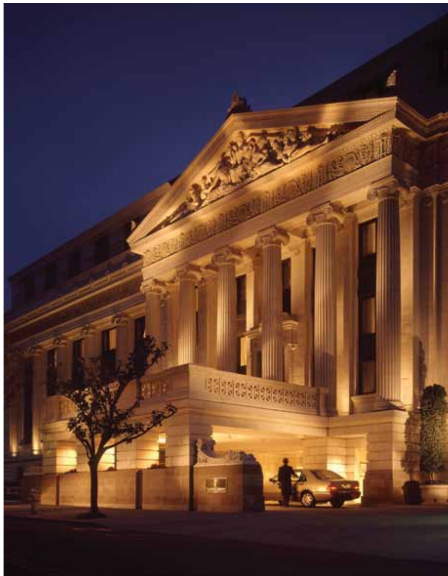
Four 60kW Capstone microturbines provide cooling, heating, and power to the prestigious Ritz-Carlton hotel in San Francisco.
